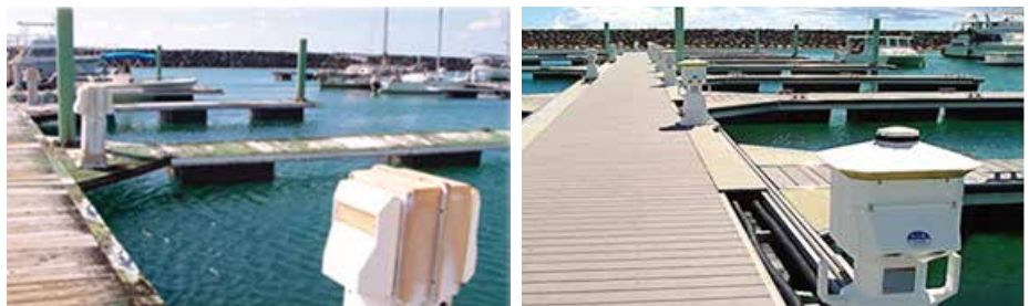
Agat small boat marina dock before and after improvement.
