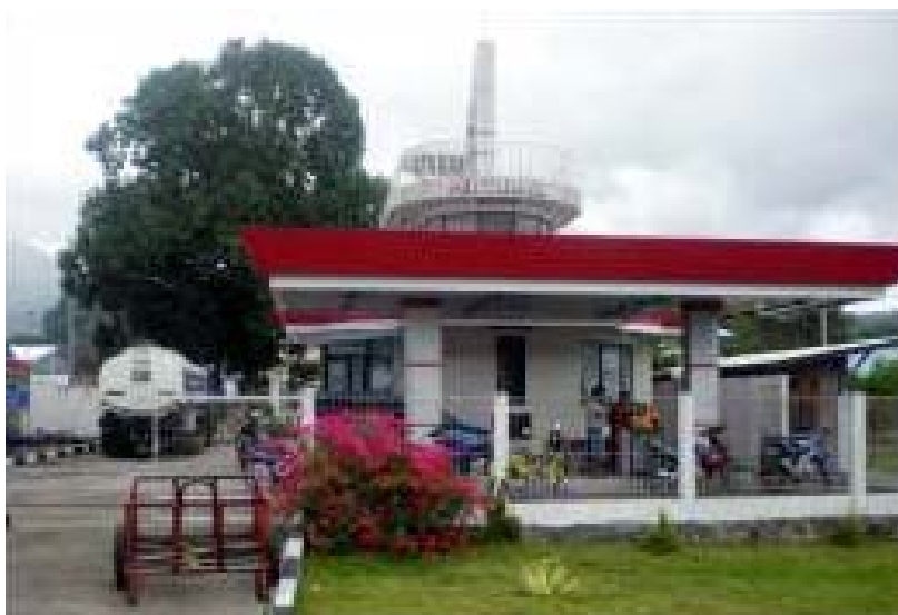
Fig. 4.2. Gasoline and diesel fuel station in Bitung OFC (Source: Indonesia Fishing Ports, 2009)
