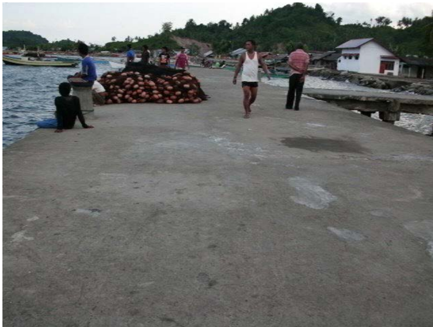
Fig. 4.12. Pier in Belang FLC (Source: MMAF 2010 o )
