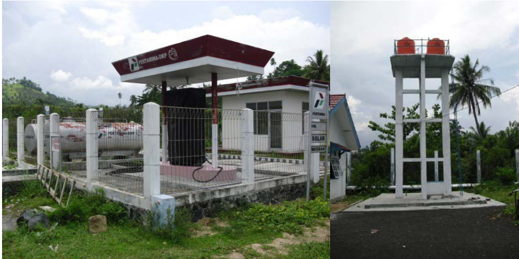
Fig. 4.7. Fueling station and water installation in Amurang FLC (Source: MMAF 2010 c )
