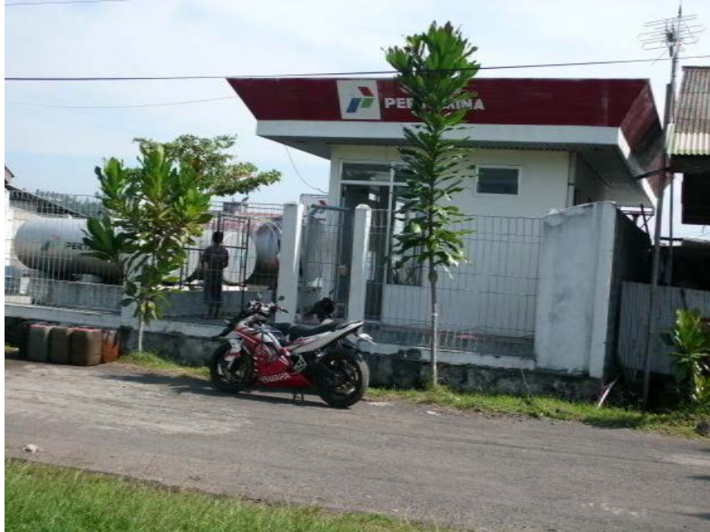
Fuel supply station
