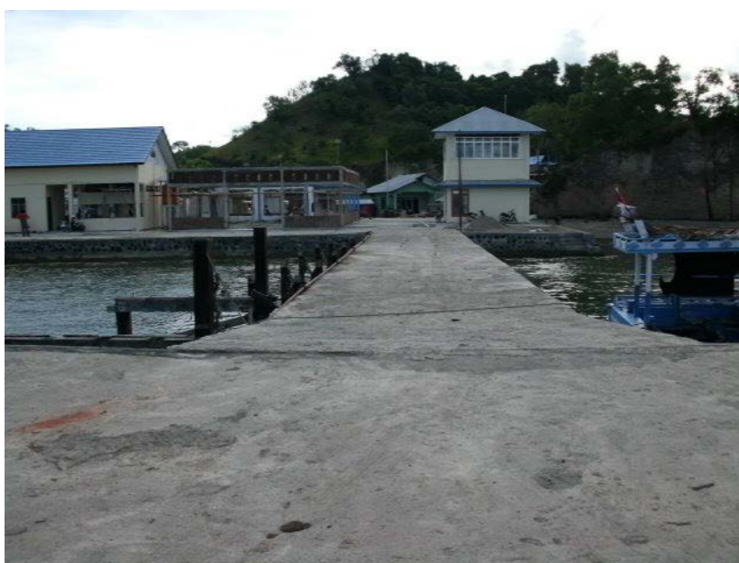
Fig. 4.9. Pier in Kema FLC (Source: MMAF 2010 c )
